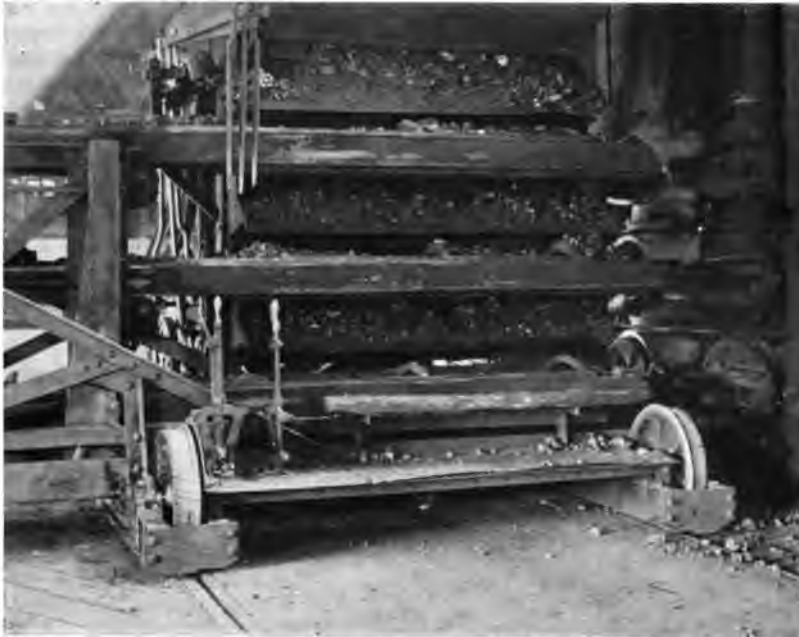
Fig. 1. Guards for Truck-Wheels of Charging Machines.*
